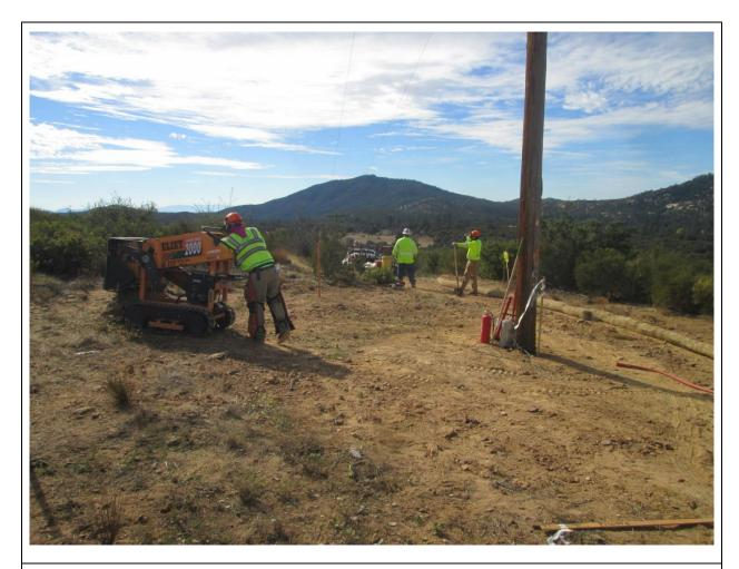
**Photo 1**: A construction crew observed clearing vegetation at Pole P176998 (C 442). The crew was observed staging the required 5 gallon backpack pump, round point shovel, Pulaski, and 2A10BC fire extinguisher, along with 100 gallons of water with pump and hose (not pictured) in accordance with Fire Prevention Matrix (off CNF land), CFPPP (MM FF-1 and APM HAZ-01), and APM HAZ-04.
