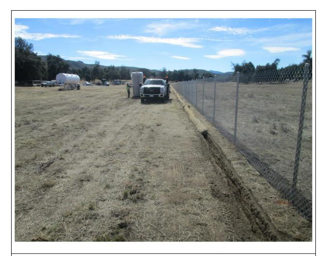
**Photo 2:** A construction crew observed installing perimeter fiber rolls at Corte Madera Staging Yard (C 442) in accordance with the project's Erosion Control Plan, SWPPP (MM HYD-1, MM BIO-7) and APM HYD-09.
