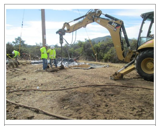
**Photo 3:** During pole hole drilling at Pole Z118044 (TL 682), drill spoils were placed on a sheet of plastic to prevent erosion in accordance with the project's Erosion Control Plan, SWPPP (MM HYD-1, MM BIO-7) and APM HYD-09.
