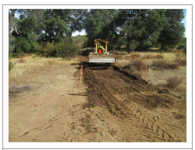
**Photo 4:** During the grading and maintenance of an existing access road near Pole P177001 (C 442), stakes were installed along the road limits to ensure grading was conducted only within approved areas in accordance with MM BIO-1.
